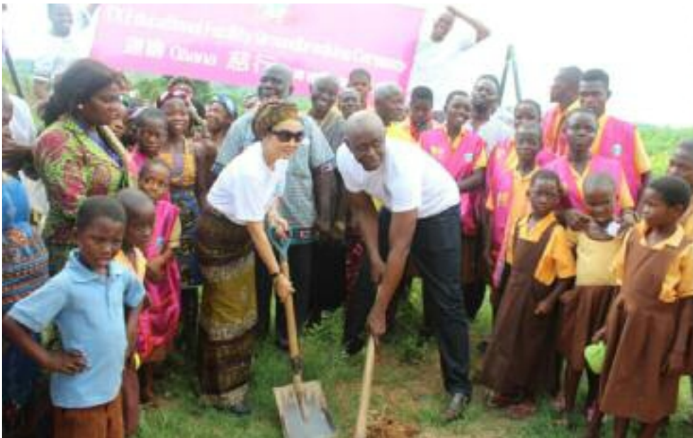
TX Foundation and AAG break ground for the construction of the facilities
