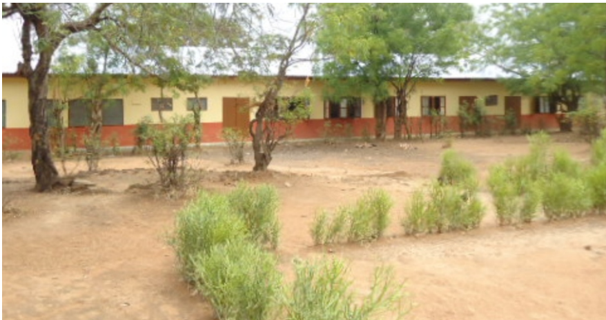
Six classroom block constructed in Challu
