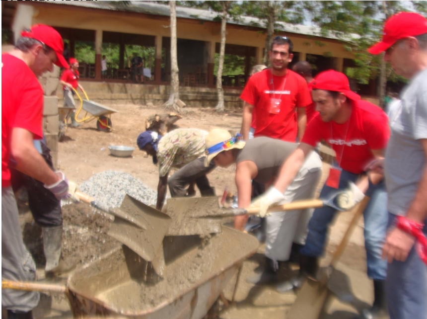
A section of Greek supporters moulding blocks at the site
